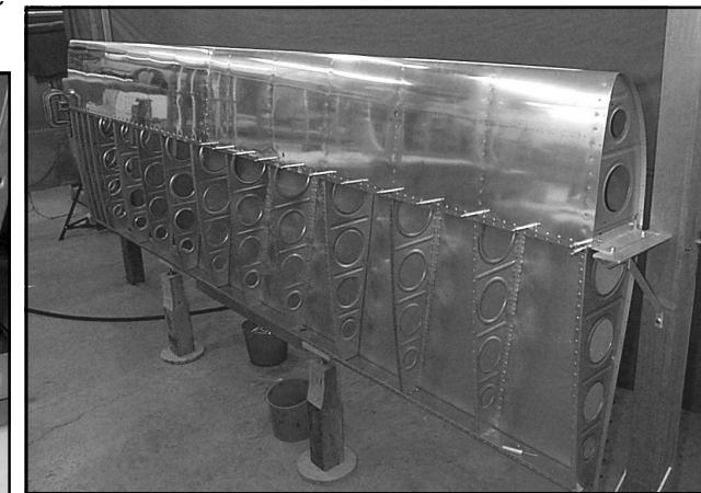
Fig. 7-5: The tank and top main skins are fitted.
