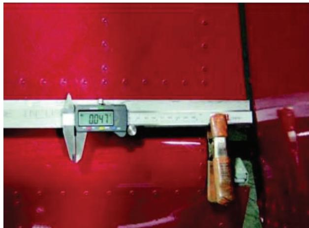
Figure 7.1: Inspect Rear Spar Doubler
