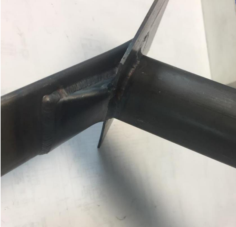
FIGURE 4: Welded assembly aft
