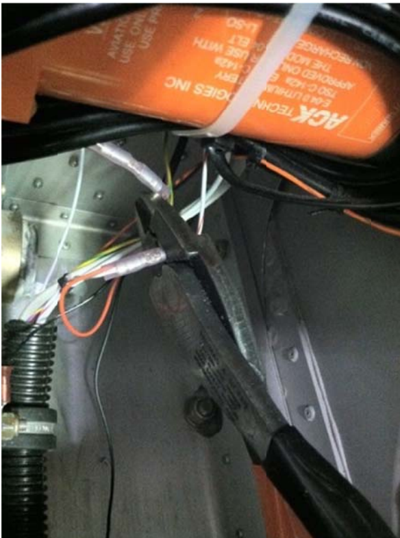
FIGURE 4: Crimping wires into the splice connector
